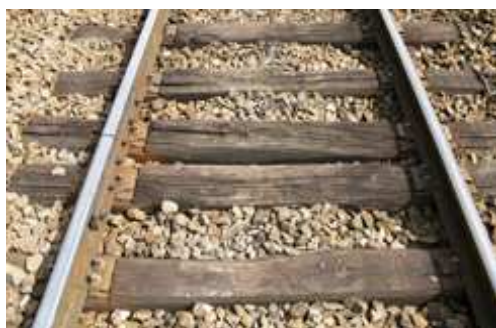
Figure 11: Rails courts sur traverses bois
